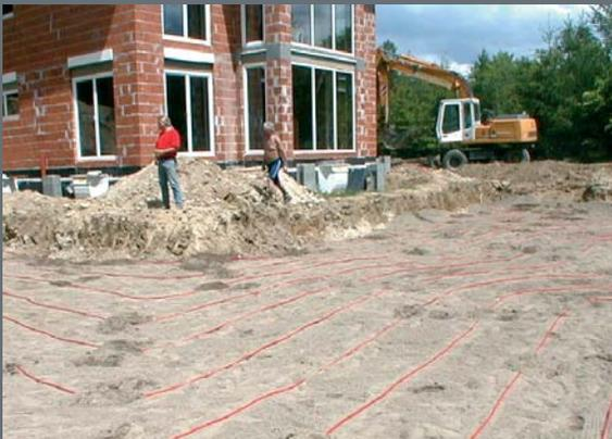
The collector area depends on the heating performance required, and the soil properties. The more dense, cohesive and moist the soil is, the more heat it can store, or make available for heating the house.
